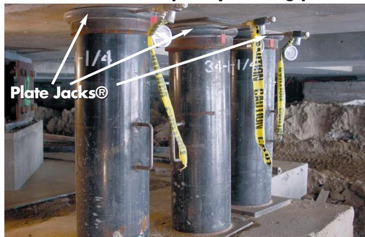
**Approximately 400 Plate Jacks®** are used as temporary shoring jacks on this project. These jacks will be re-formed and re-used multiple times during the life of the project.
